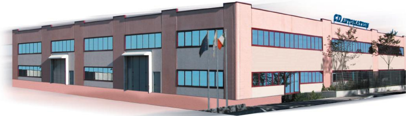
Our facility in Legnano for thyristor unit production
